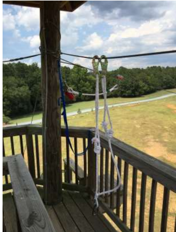
Completed zip line rigging at Belk.
